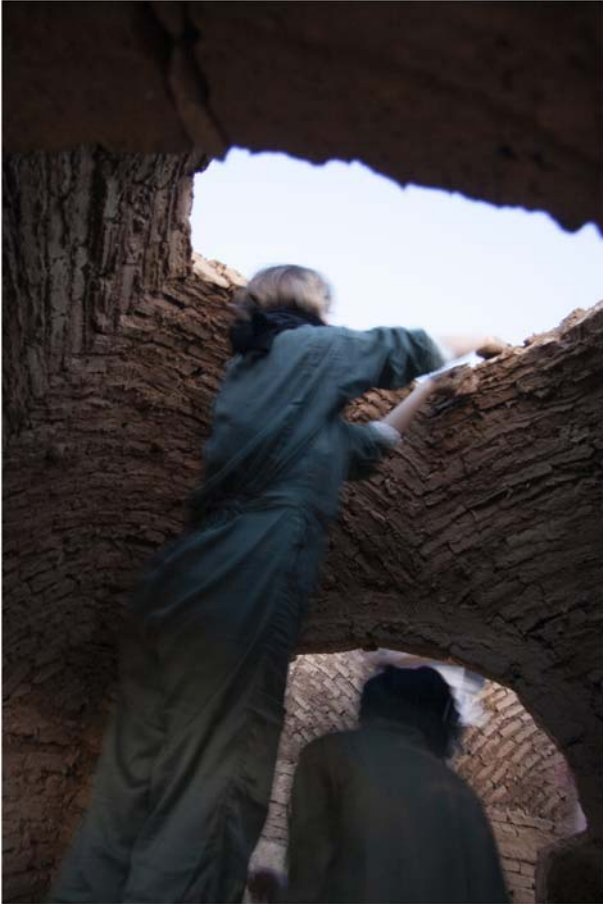
Figure 12. The making of a squinch vault during a workshop in February 2018.
