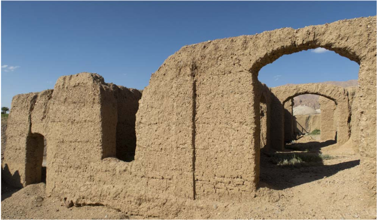
Figure 5. Incomplete house that was being built at the time of the Tabas earthquake by Ostad Habib.
