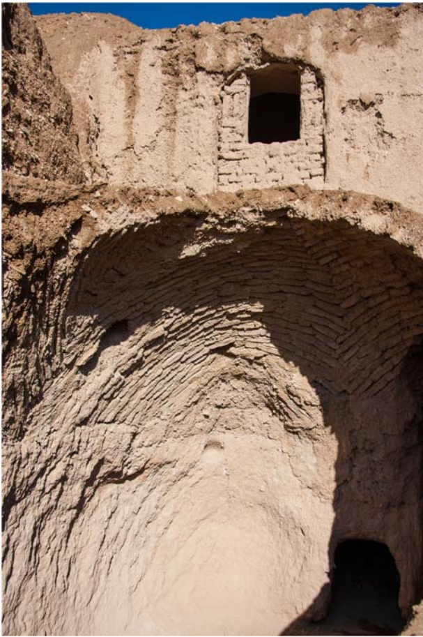
Figure 2. A hand-carved room ( dastkand ) covered with a vault.
