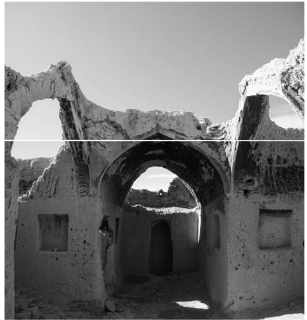
Figure 4. An abandoned 4-sofeh pattern house, photo collage.
