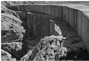
Fig. 6. The Concrete Dam Next to the Historic Kobar Dam ( https://mapio.net/pic/p-64824407/ , 2017)
