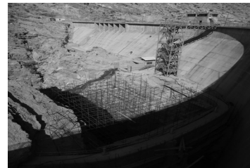
Fig. 7. Concrete Dam Next to the Historic Kurit Dam (Tabas, 2012)
