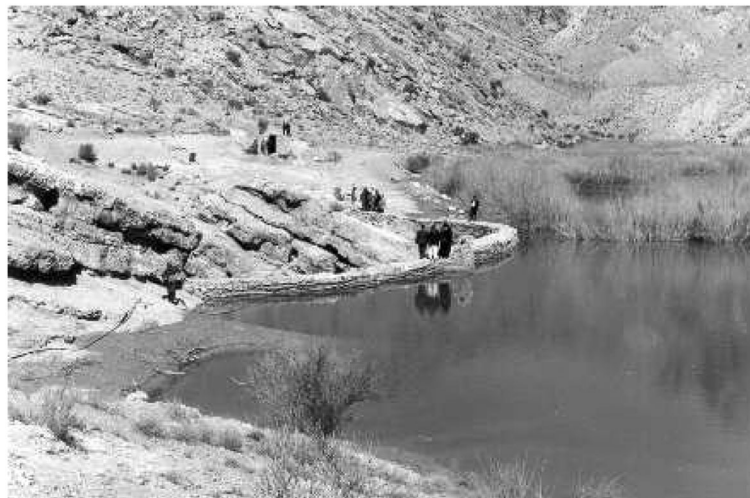
Figure 5. A view of the Kurit Dam showing the arch geometry, March 1998 (the top of the water intake is shown near the centre of the arch and the operating room can also be seen)
