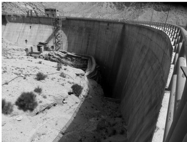
Figure 8. The old and new Kurit dams (2013)
