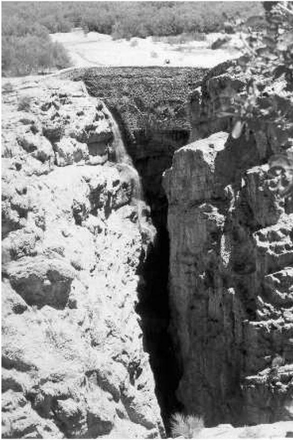
Figure 2. The Kurit Dam (May 1999)
