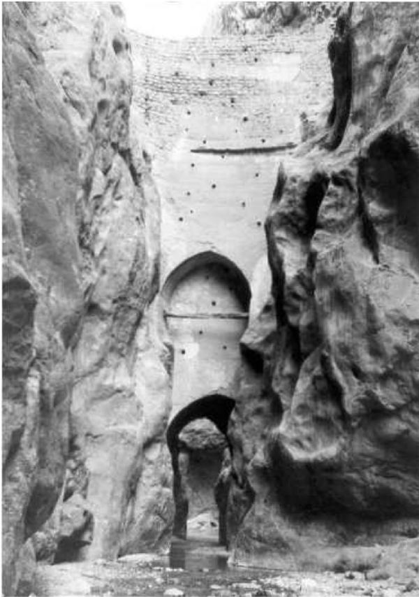
Figure 3. A 25-m high Abassi flood retention dam near Tabas, Iran, with similar bridge diversion system
