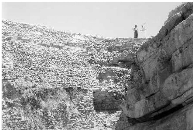
Figure 4. A view of the dam from downstream indicates the use of different materials in the stage construction (the hole near the abutment was intentionally made when the intake was blocked)
